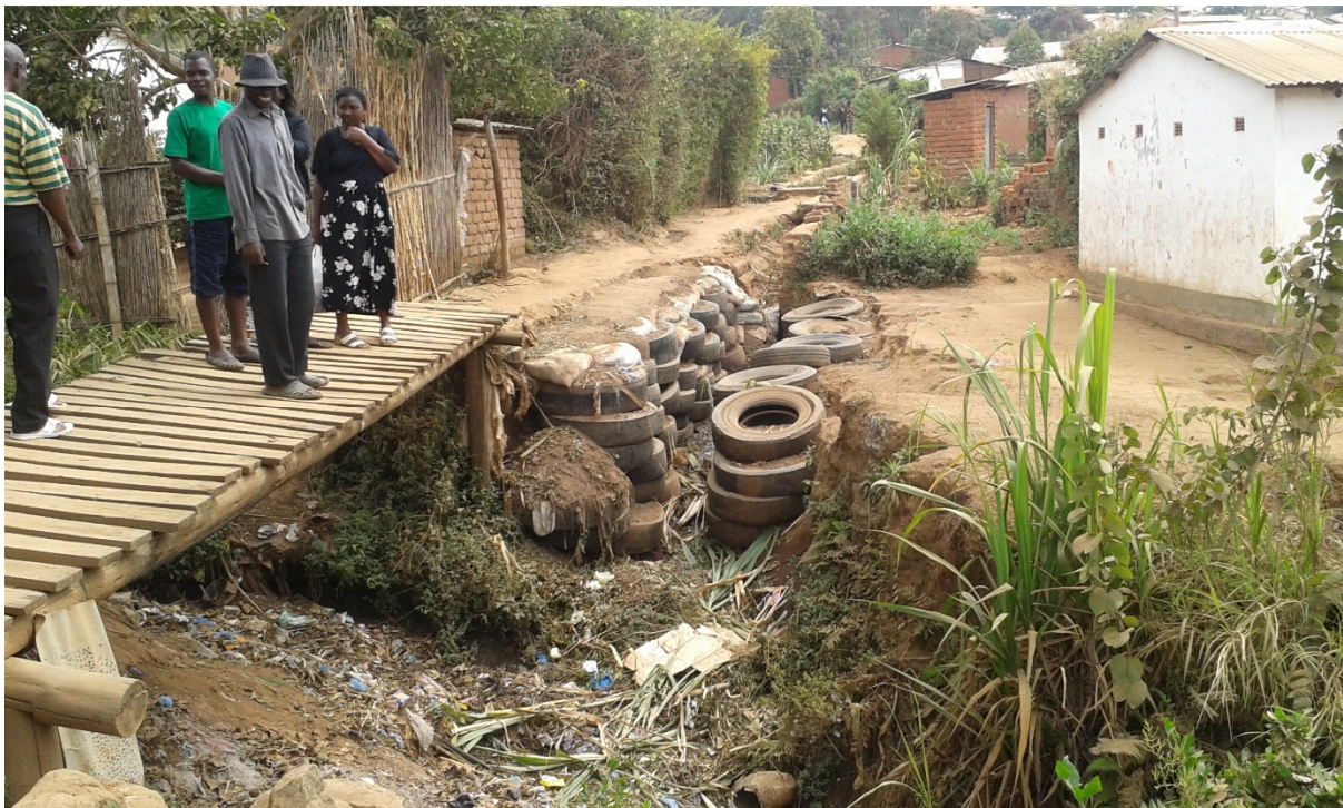
Figure 6: Existing bridge and adjacent gully, showing erosion protection
