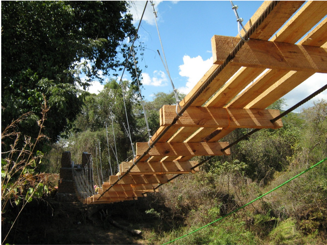
The bridge as-built in 2007 – view from left bank
