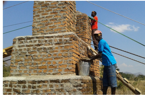
Figure 8: Skilled builders re-pointing the towers
