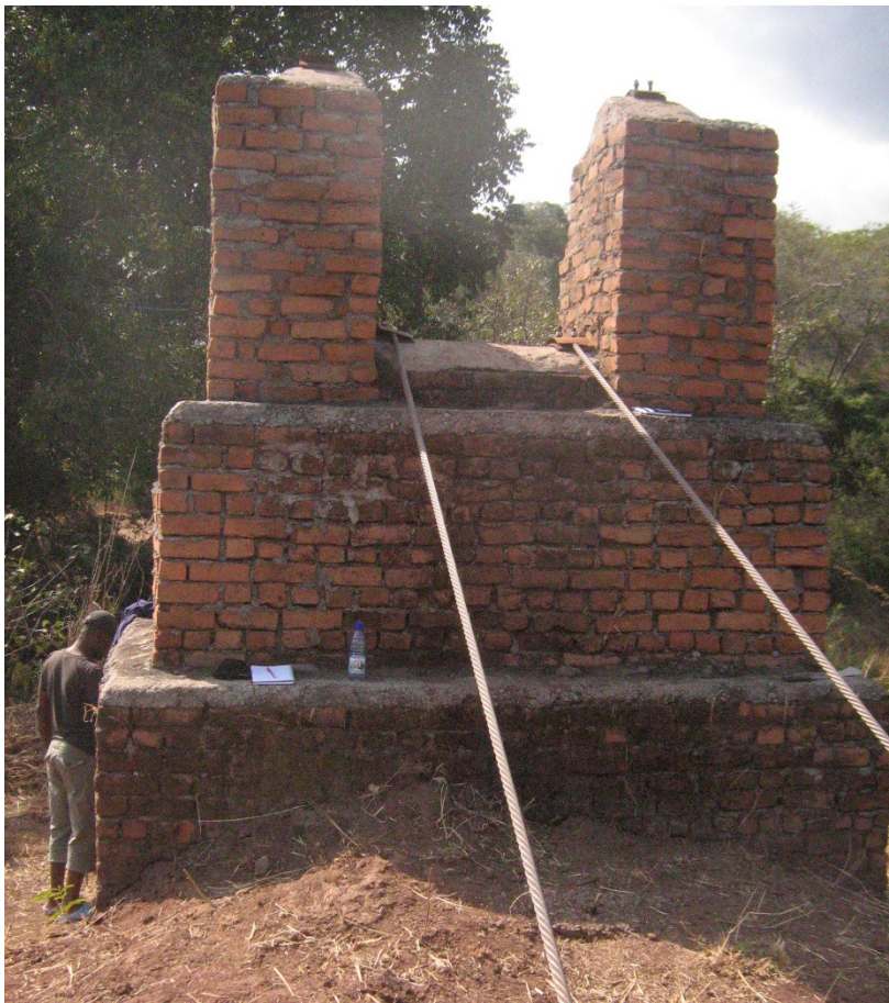
Tower generally in good condition
