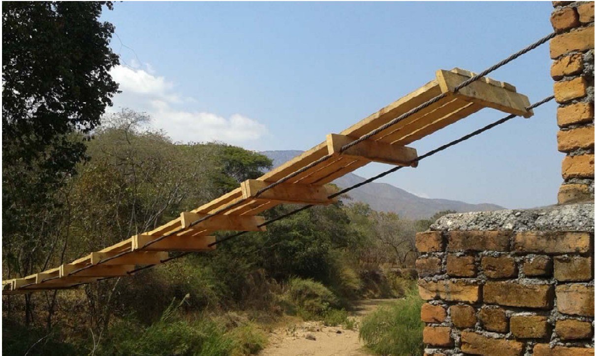
Decking units replaced
