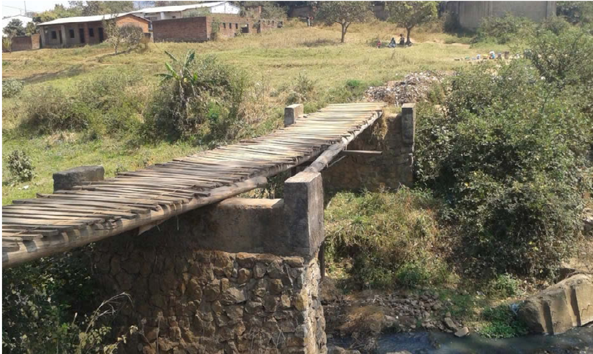
Figure 3: Chiwembe Bridge, viewed from the left bank
