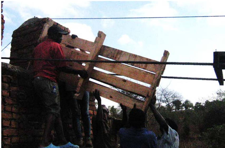
Figure 14: Lifting a new decking unit into place
