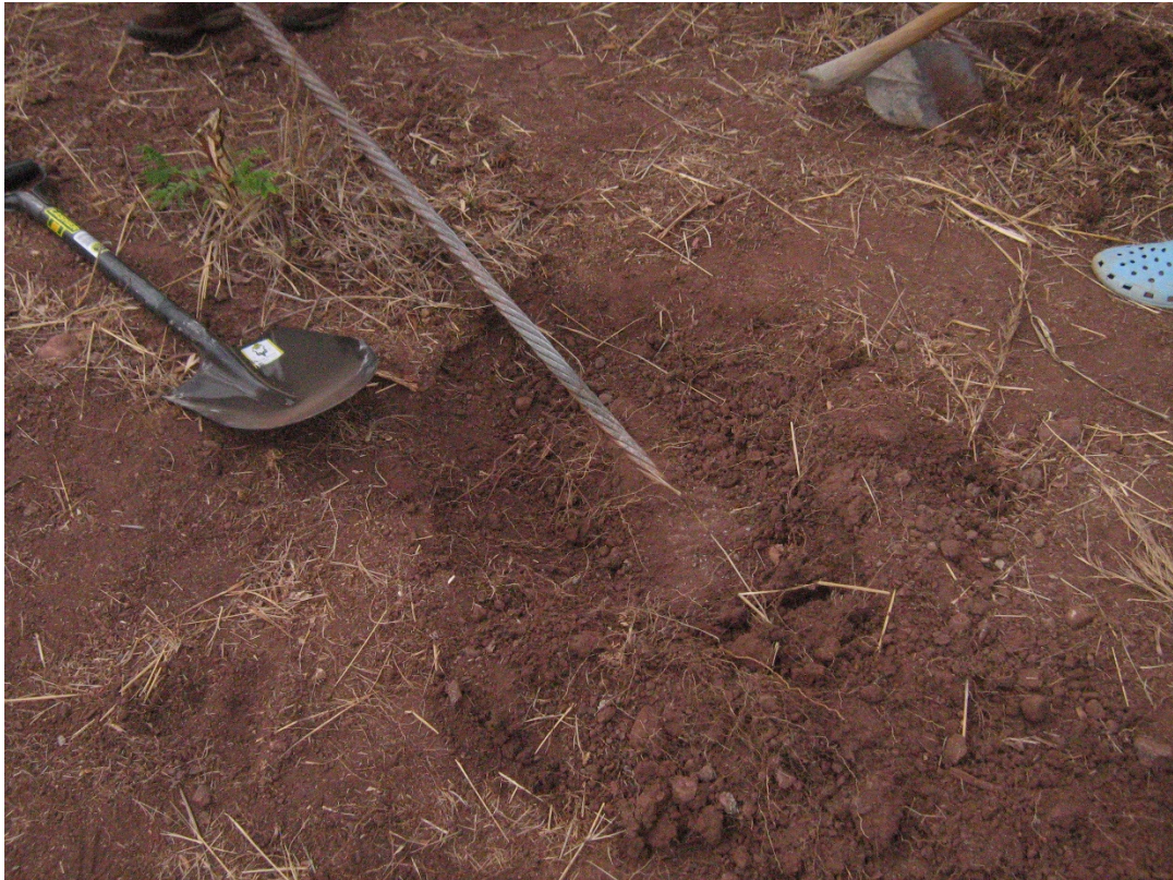
Main walkway cable in good condition
