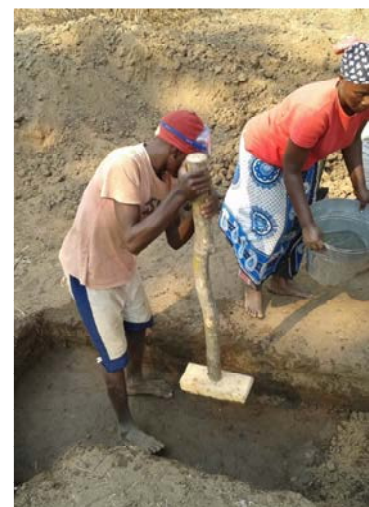
Figure 12: Compacting embankment material using a homemade rammer
