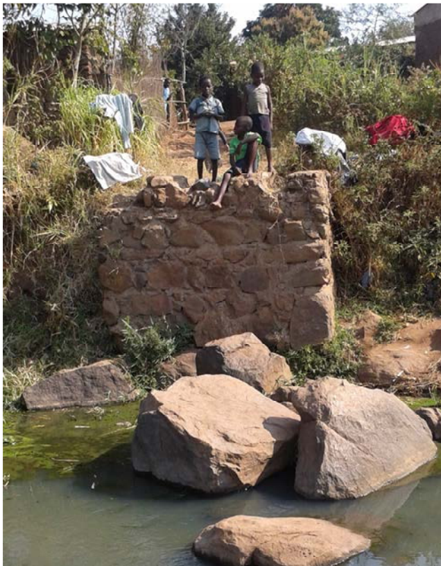
Figure 2: Existing crossing point from left bank, showing stepping stones and right abutment
