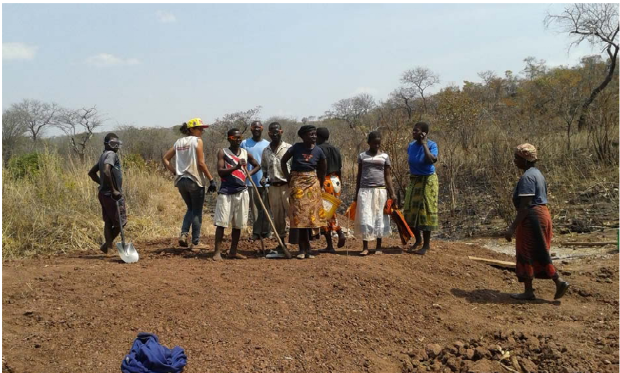
Compacting embankment to 0.5 m above ground level
