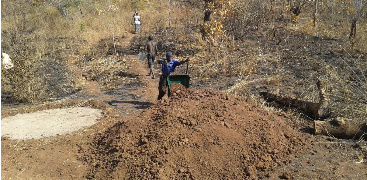
Figure 13: Stockpiling soil for embankment construction
