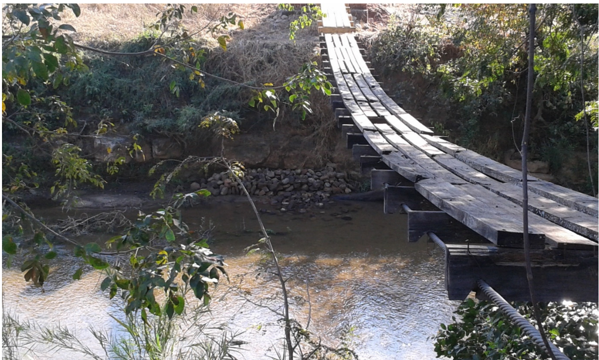
River bank protection on left bank
