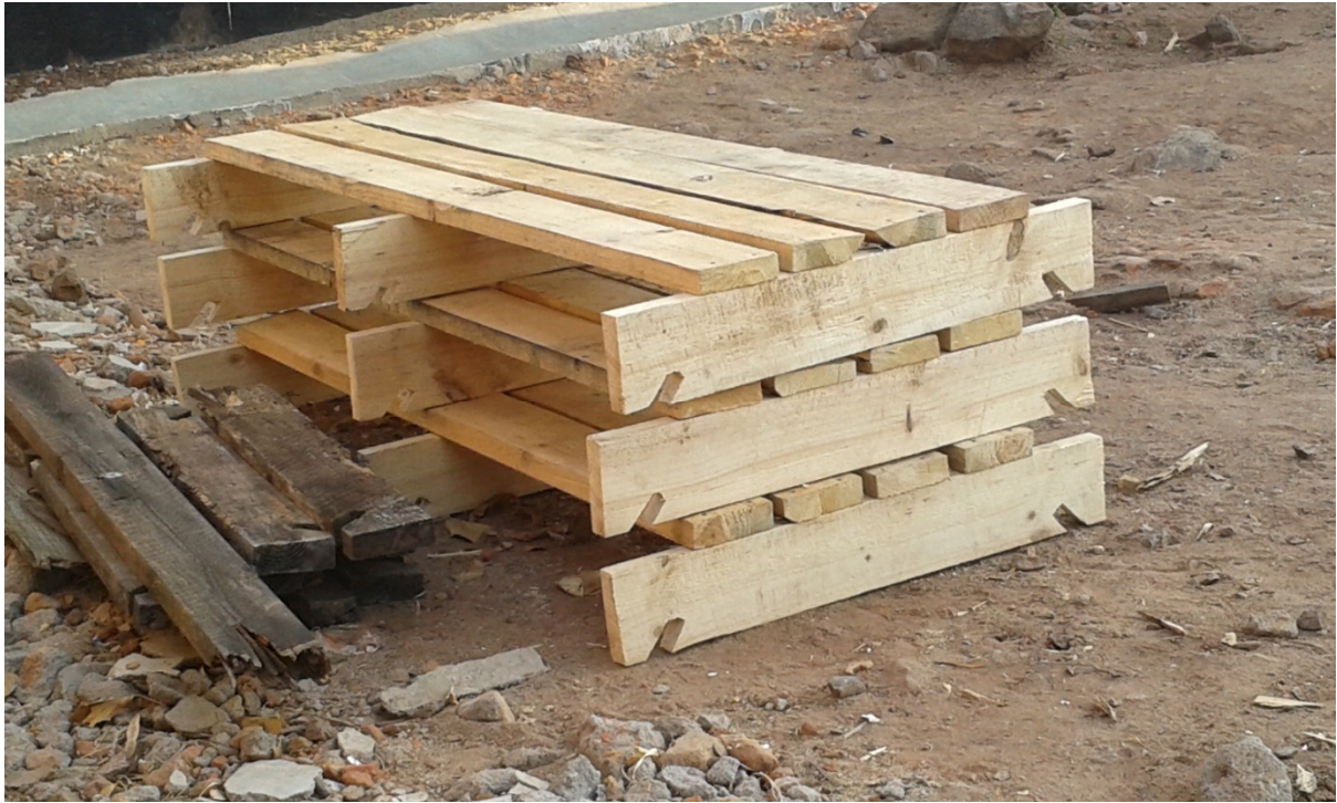
Replacement decking units
