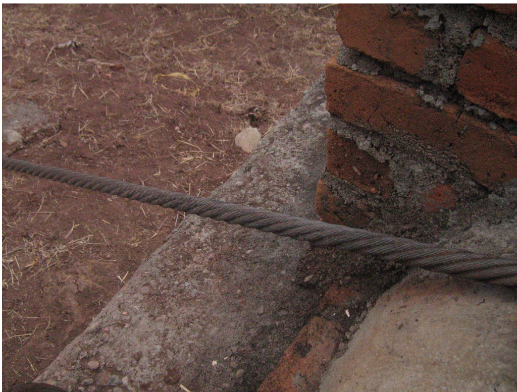
Main walkway cable in good condition
