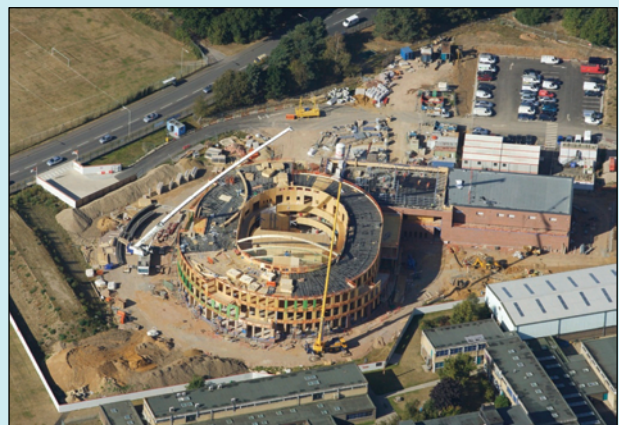
Figure 10: Aerial view of the Open Academy during construction.
