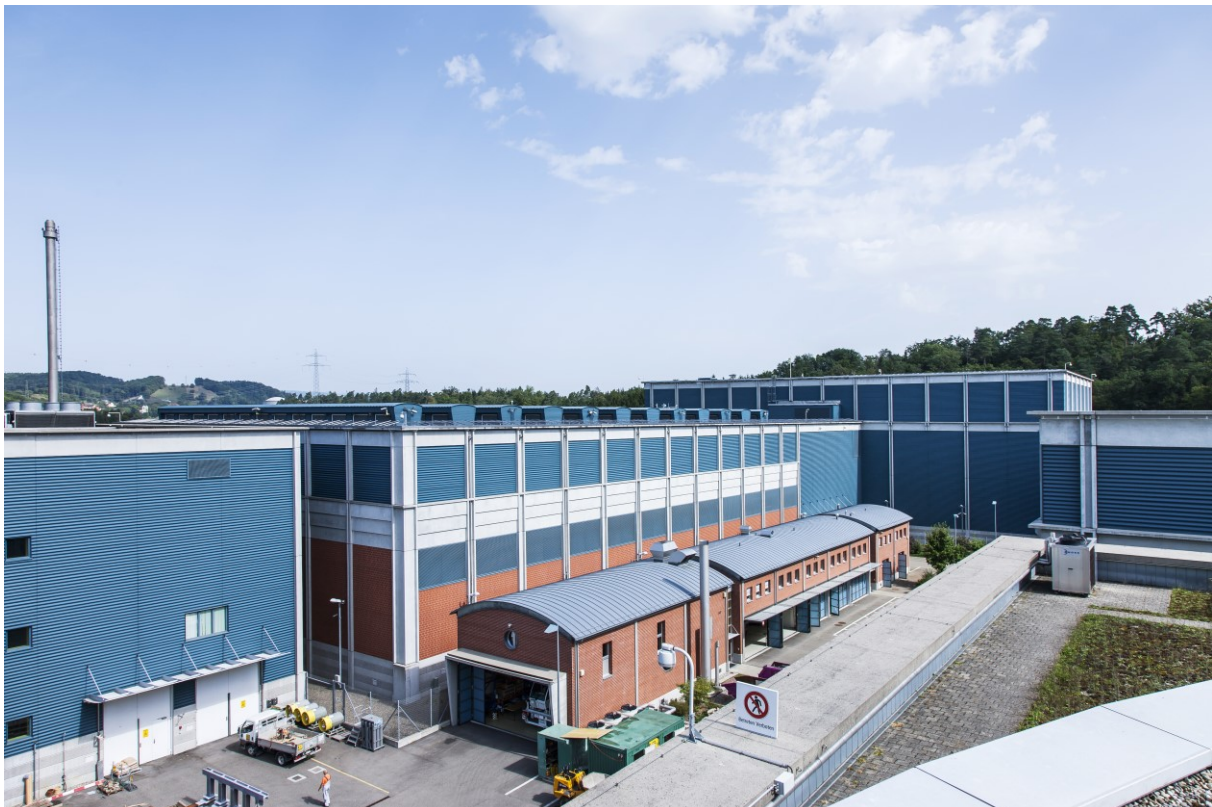
Figure 4: Central Interim Storage Facility of radioactive waste (ZZL) in Würenlingen. The facility is operated by the utility-owned company Zwiilag (Photo: ENSI).
