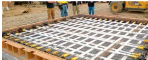
Figure 1: Test Slab Fabrication with Post-tensioning and Reinforcement
