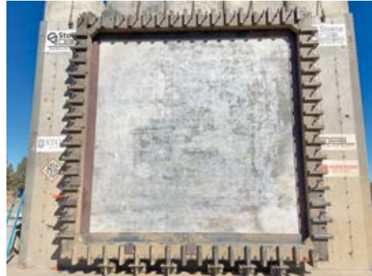
Figure 7: Installed Panel within the Stiffer Frame Set-up No. 2
