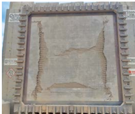
Figure 10: Front Face Slab Scabbing in Test 6
