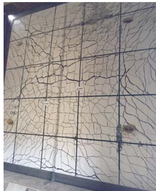
Figure 9: Highlighted Cracking Pattern on Back Face in Test 3
