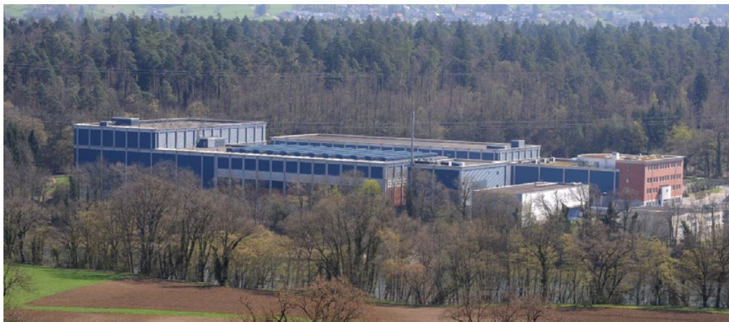
Figure 3: Central Interim Storage Facility for radioactive waste (ZZL) in Würenlingen. The facility is operated by the utility-owned company Zwilag (Photo: ENSI).
