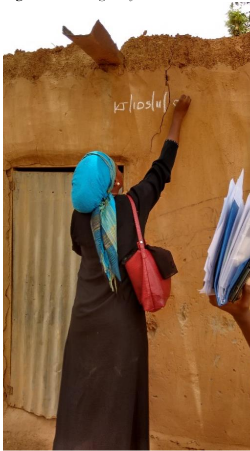
Figure 2: Marking out of children's reach
