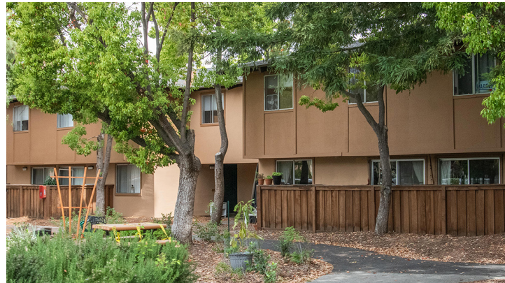
Escondido South Two-story Low-Rises, Exterior
