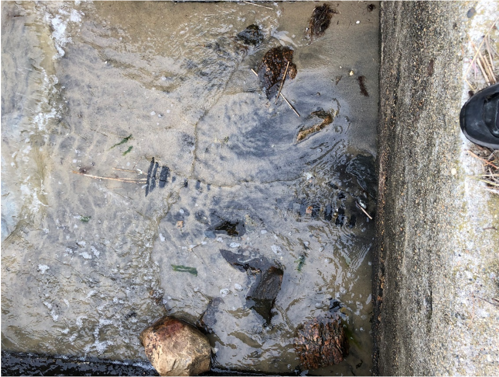
Figure 3: Source 8-5-508, 15” pipe (filled with sand, no flow in 2019).
