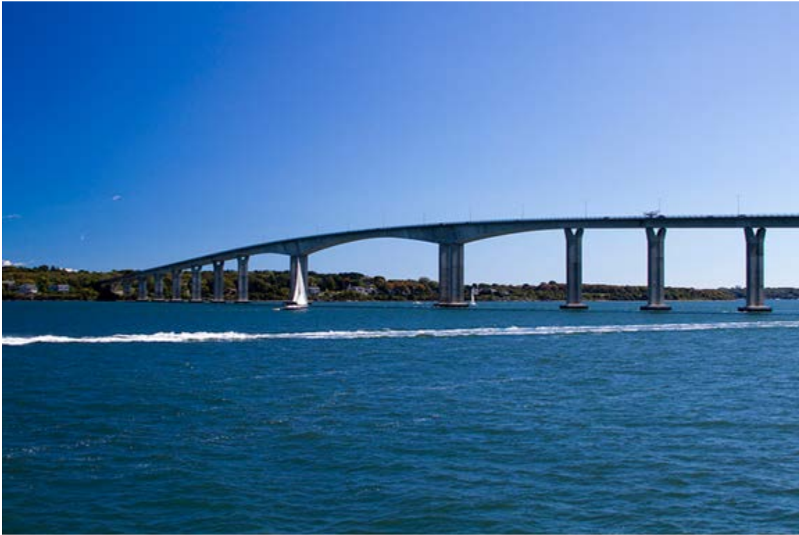
Jamestown Bridge West Passage
