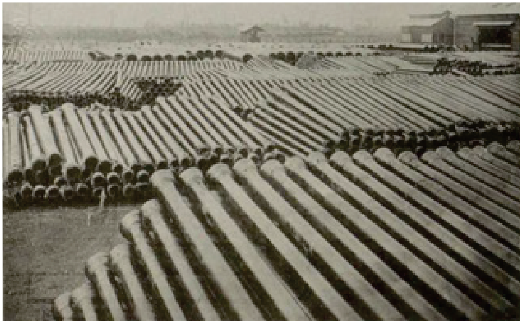
Figure H.2: Cast-iron pipes of the modern water-supply system ( Chutetsukan )
