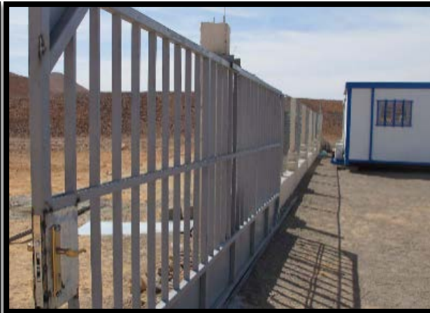
CW elimination & physical security, Libya
