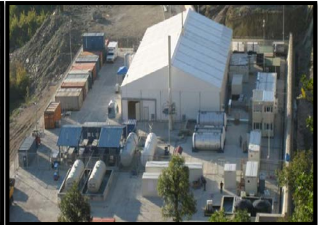
CW destruction facility, Albania
