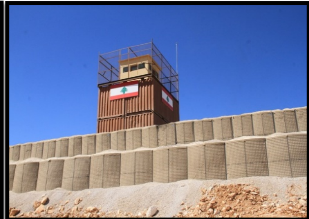
Land border surveillance tower, Lebanon
