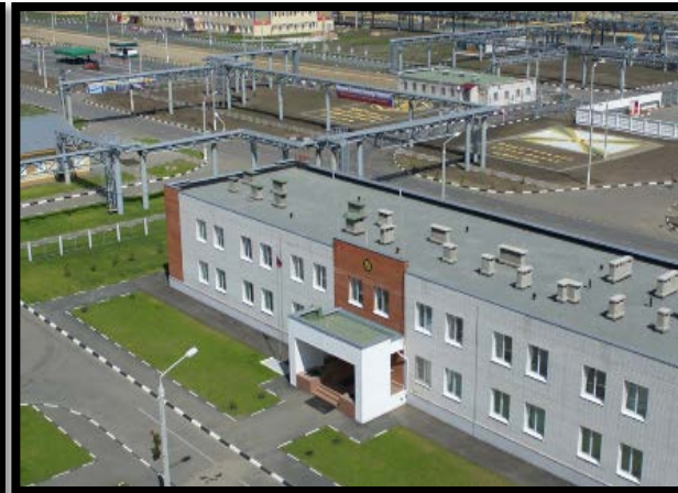
CW elimination & destruction facility, Russia
