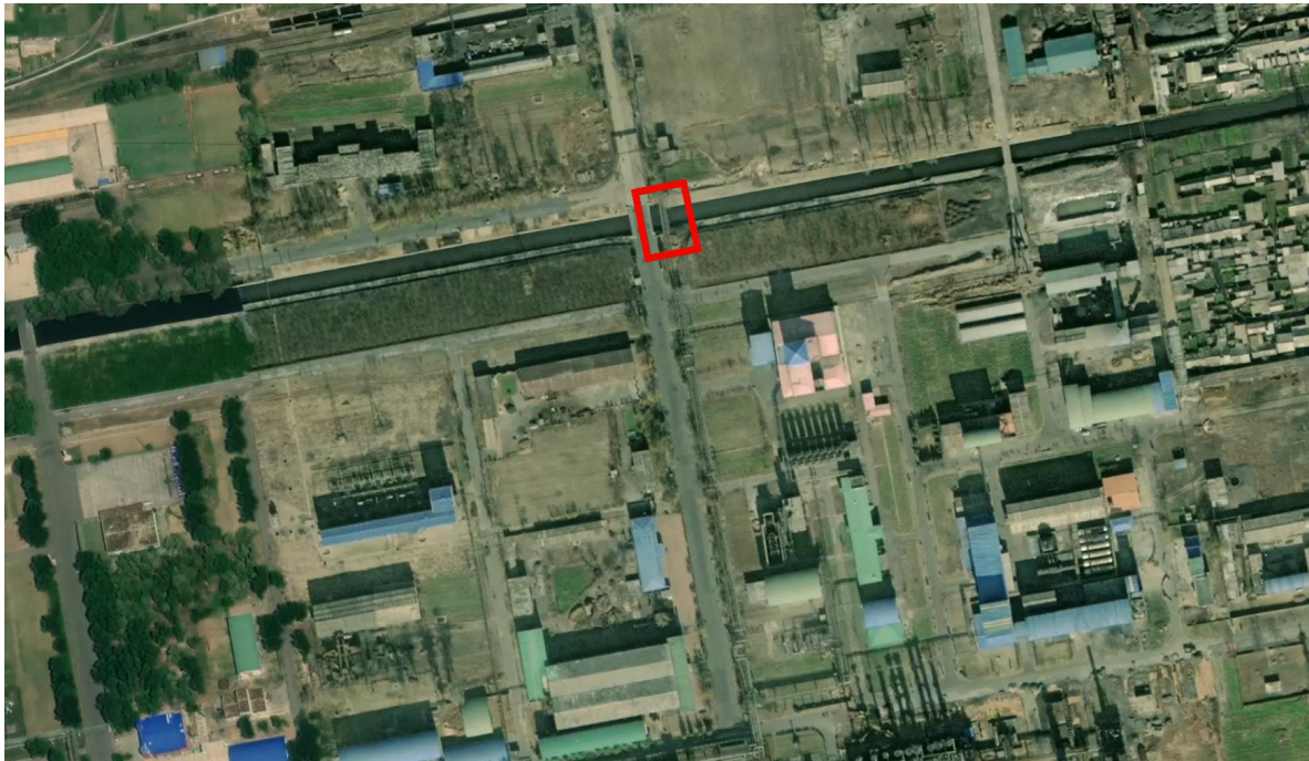
Figure 5: Pipework Connects the Southern and Northern Parts of the Complex
