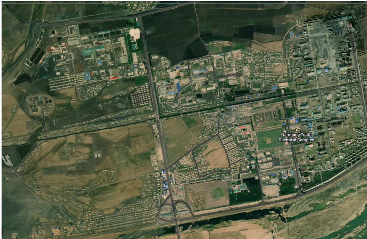
Figure 1: Overview of the Namhung Youth Chemical Complex
