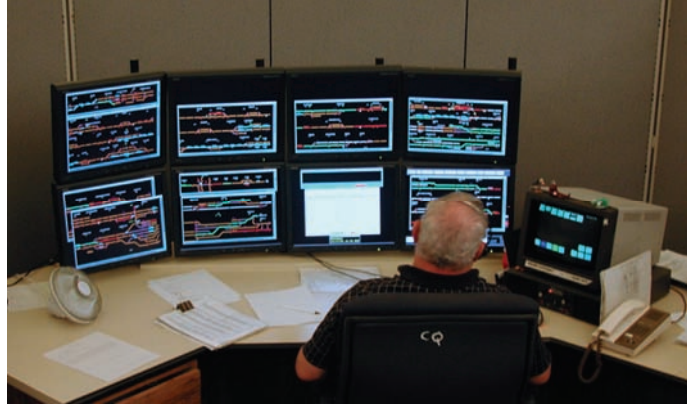
Figure 6-2. CSXT Train Dispatch Center
