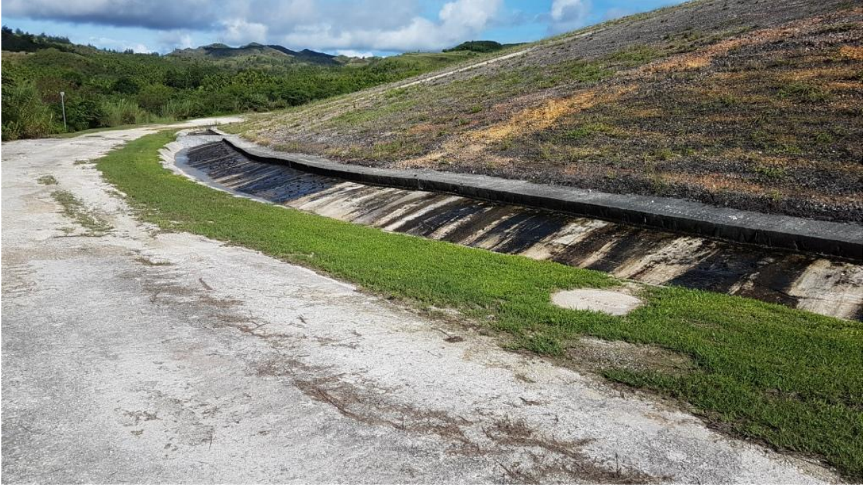
1. East PLCT MH-9 cover looking in a southwesterly direction.
