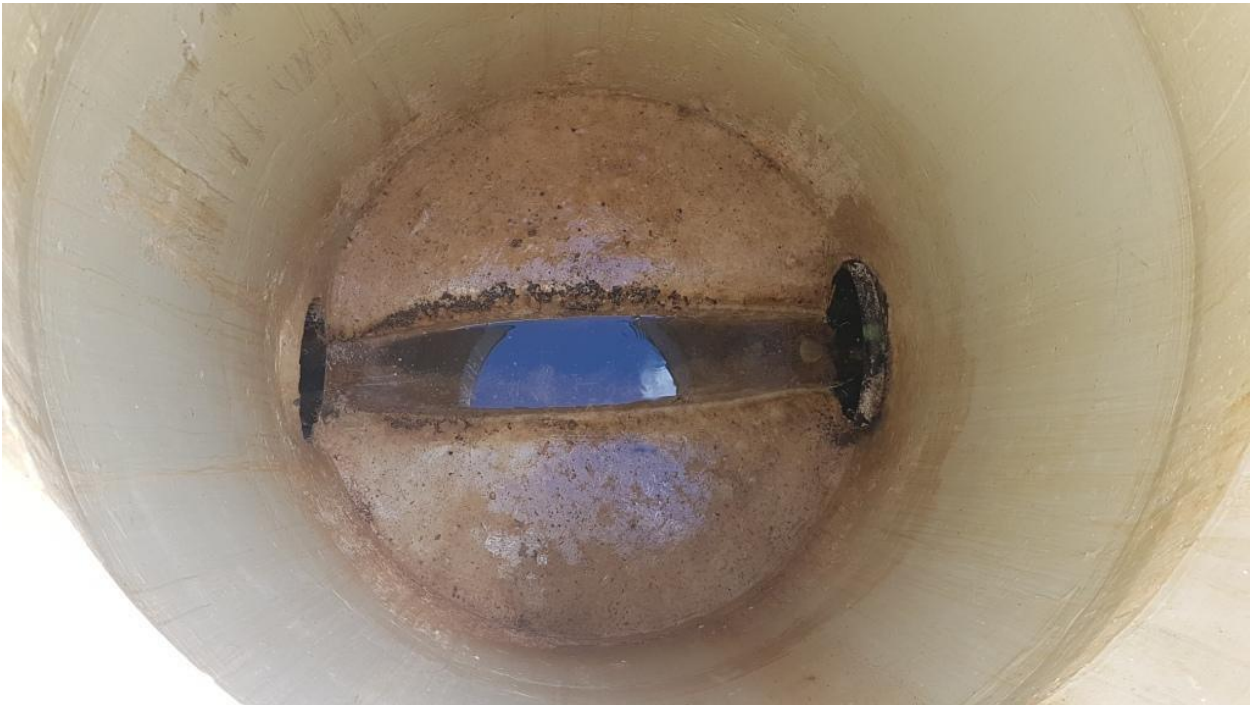
4. West PLCT MH-11 invert.
