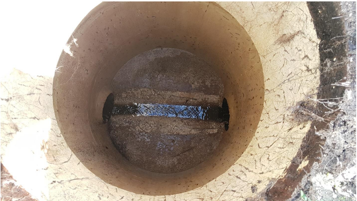
2. East PLCT MH-9 invert.
