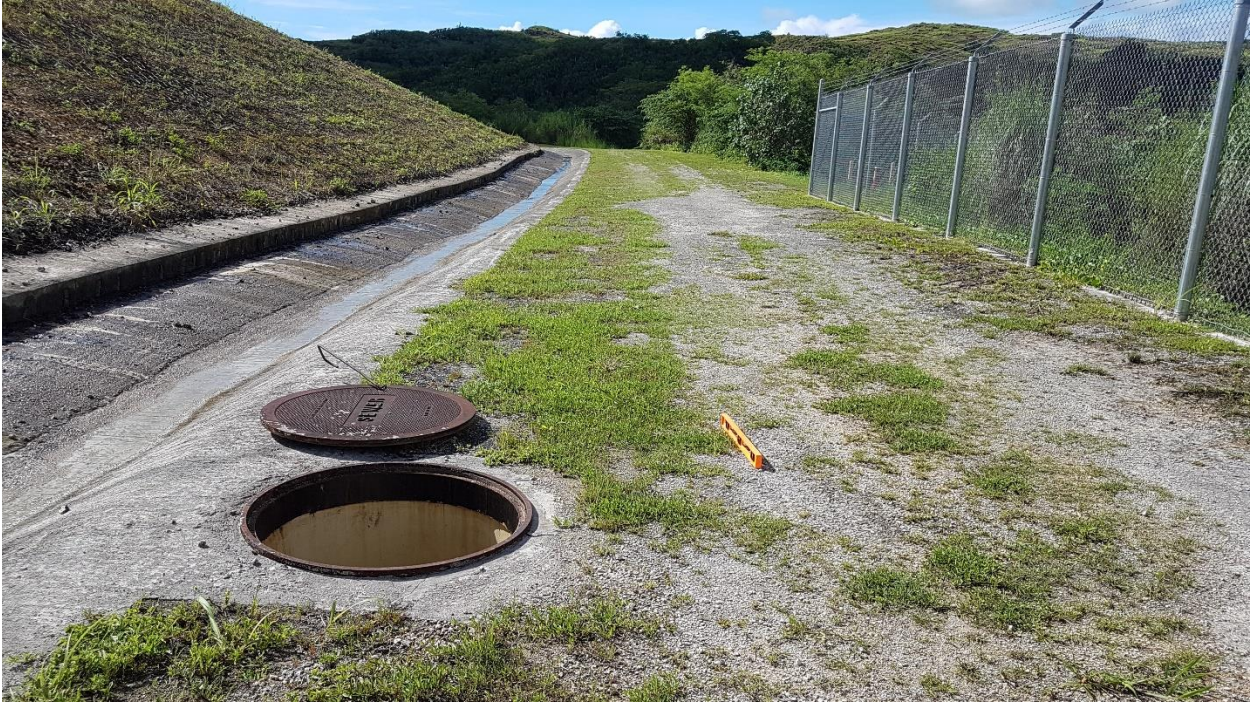
3. West PLCT MH-11 cover looking in a southeasterly direction.
