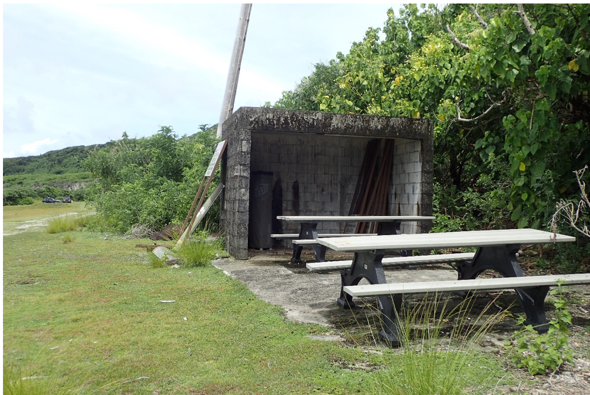
Photo 4. Cement/personnel bunker (looking east)
