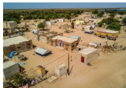
View of ville with the electric installations, region of Saint Louis, Senegal. 31.01.2019.
