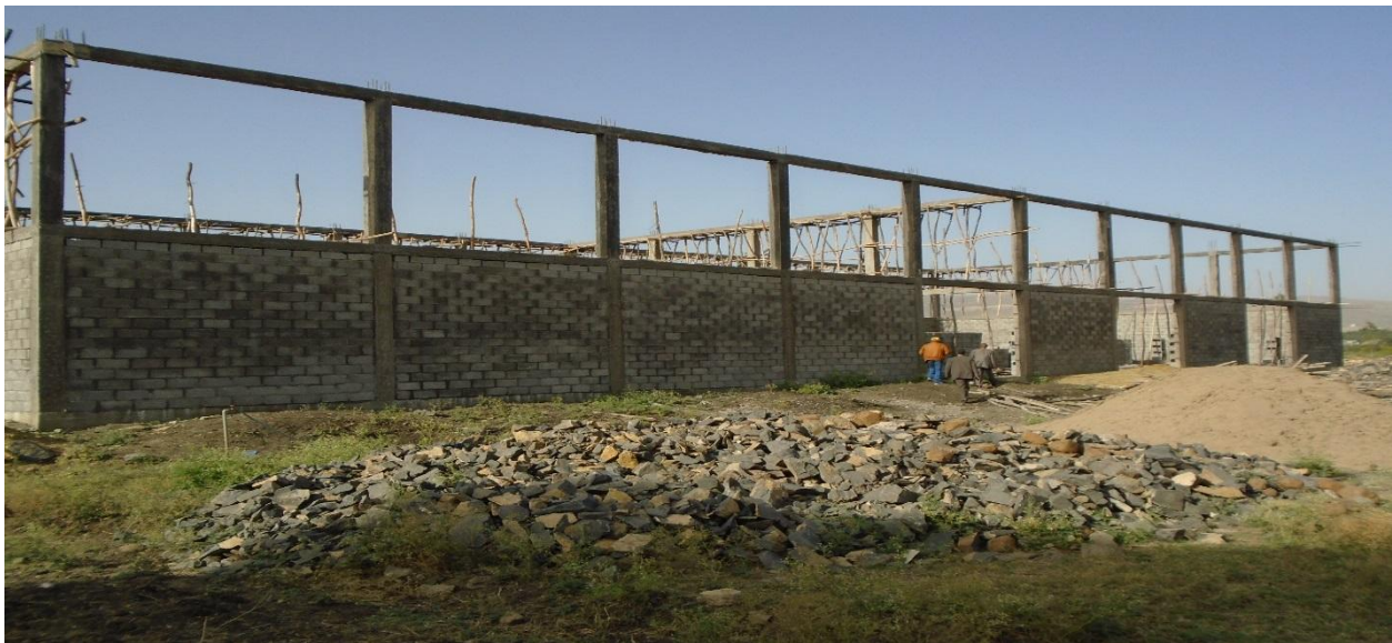
Photo: The new factory site with construction work in progress
