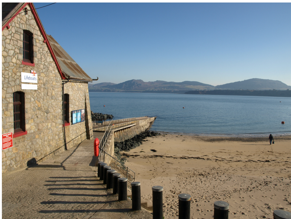
Figure 8. The RNLI slipway and the three associated RNLI buoys. Image: J. Egerton
