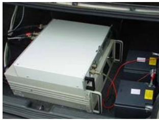
Fig.4 - TAG and batteries supply installation for van experiment.
