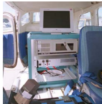
Fig.3 – TAG installation for skewed redundant configuration.
