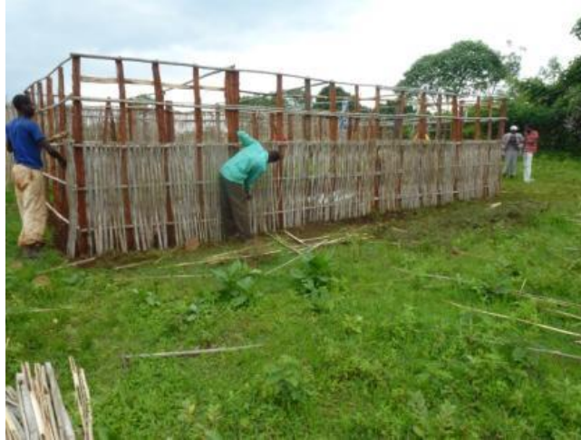
FIGURE 2. SOAK PIT FENCE MAINTENANCE USING LOCAL MATERIAL (BAMBOO), BEGI DISTRICT
