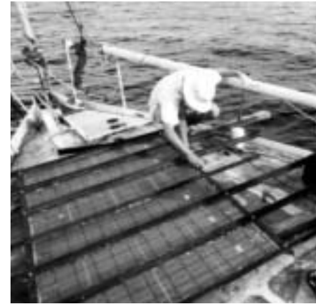
Work on the photovoltaic raft
