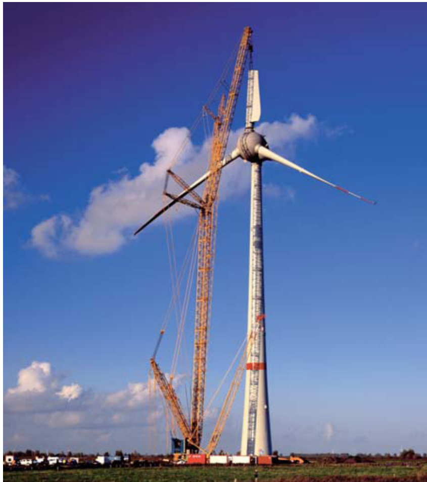
Figure 1 – An Enercon E-126 plant under construction, using a gigantic, powerful crane.
