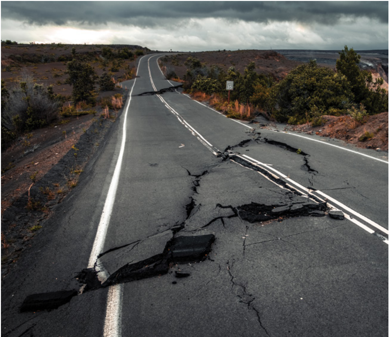
Crater Rim Drive in the Hawaii Volcanoes National Park shows damage caused by the earthquake and eruption of the Kilauea volcano in May 2018. Needed repairs in the park, such as restoring paved roads, totaled $92.7 million in 2018. Dudarev Mikhail/Shutterstock
