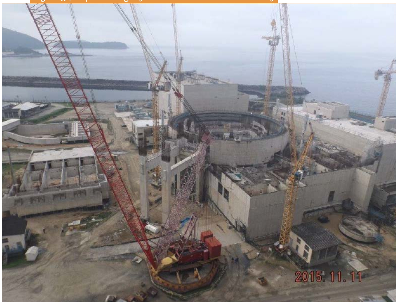
Figure 47 | Suspended Angra-3 Construction Site in November 2015
