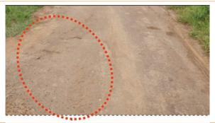
3: Poor: Poor shape and seriously restricts water to run off the road surface into the roadside drains; severe erosion of shoulder
