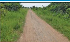
2: Fair: Uneven shape, but allowing most water to run off the road surface into the roadside drains; some erosion of shoulder
