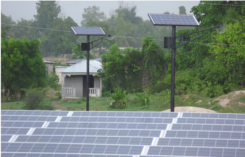
Solar panels on the roof and on street lamps capture sunlight for electricity and lighting.
