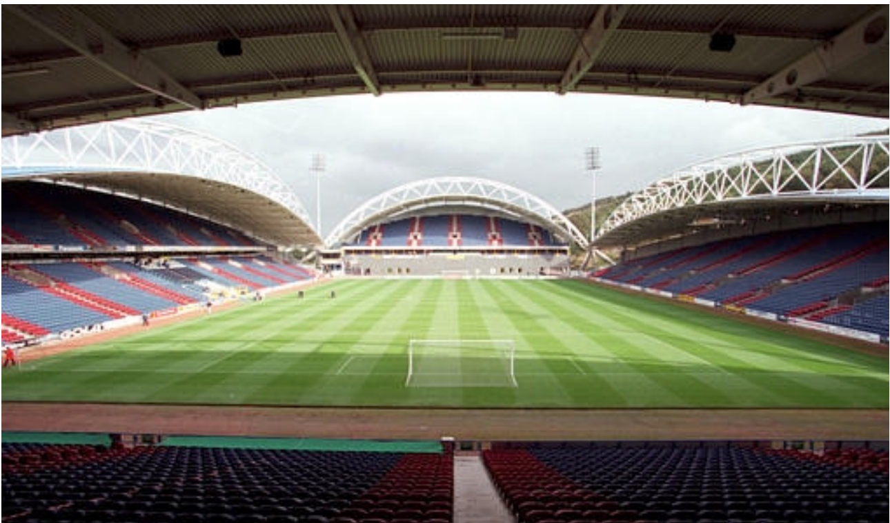
Alfred McAlpine Stadium (Huddersfield Town FC/Huddersfield /Sheffield RLFCs)
