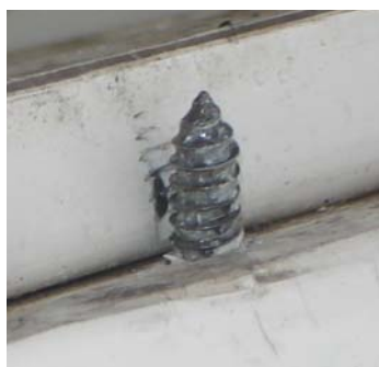
One of the four self tappers holding the console on!
