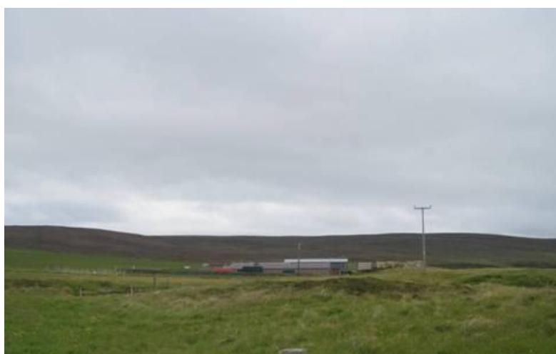
Figure 24: EMEC Substation for the Tidal Test site on Eday, Orkney (Photograph courtesy of Orkney Islands Council)
