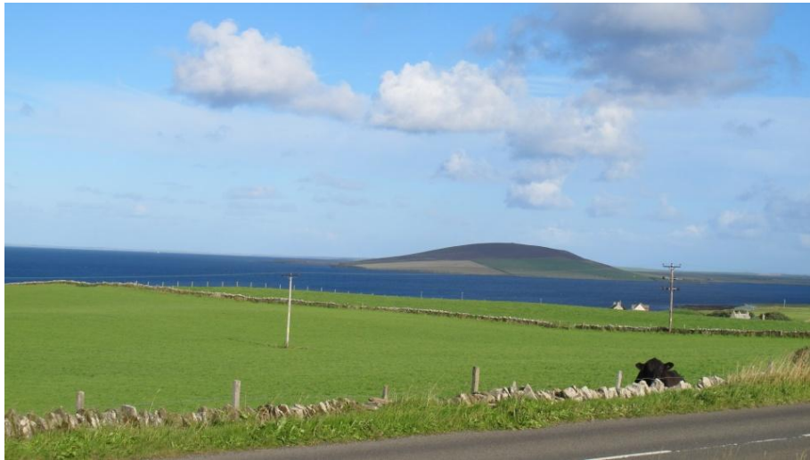
Figure 14: 33 kV Overhead Lines on Orkney
