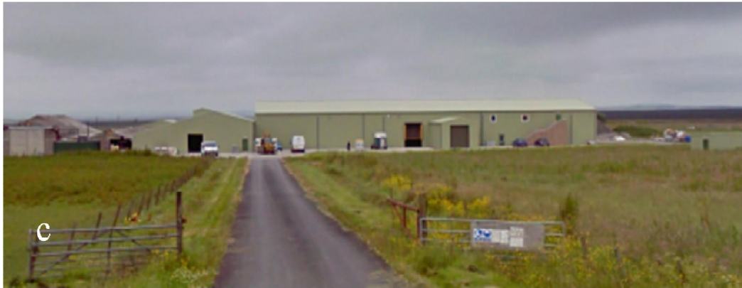
Figure 11: Halkirk Industrial Building in Caithness Landscape est. 12 m Height. (Photograph courtesy of SSE)
