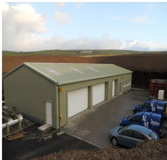
Figure 12: Aquamarine Power's Oyster 800 Building and Compound for their 2.4 MW Deployment at the EMEC Billia Croo Site (Photograph courtesy of Aquamarine Power Ltd)
