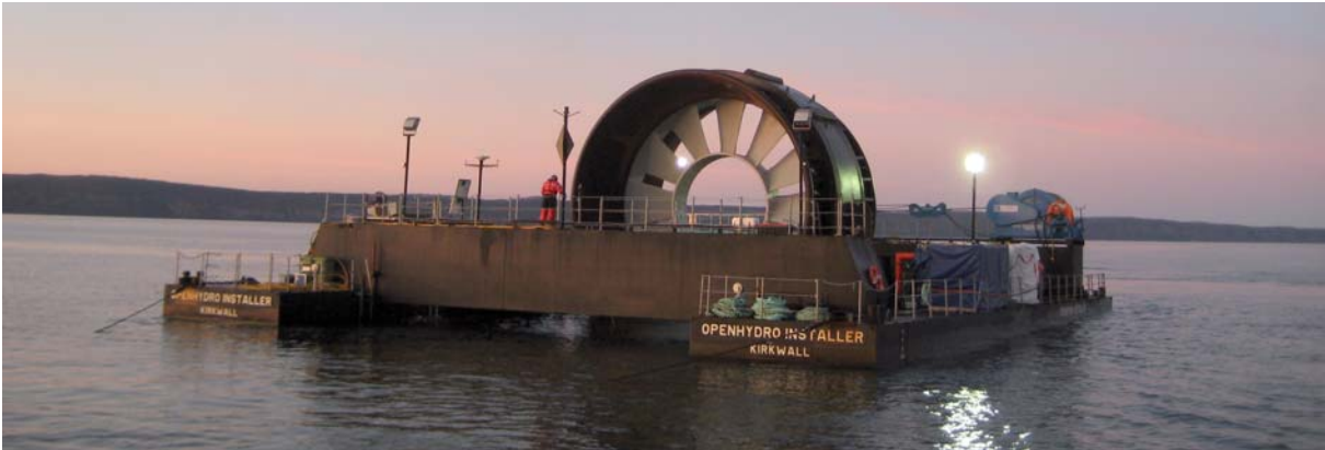
Deployment of OpenHydro turbine, OpenHydro
