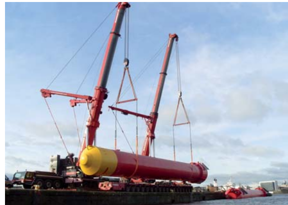
Pelamis module being lifted, Pelamis Wave Power
