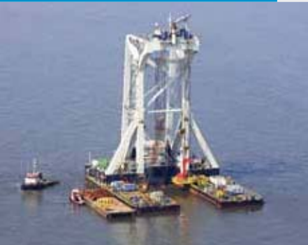
The Svanen vessel (here working at Sheringham Shoal) can lift 8,700 tonnes.
