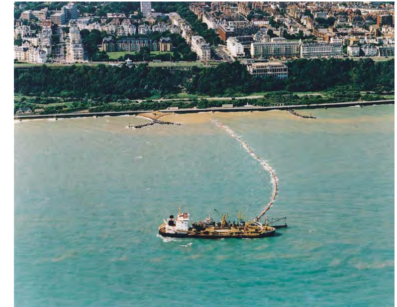
Figure 13.1: An aggregate dredger pumping sand to shore to supply a beach replenishment scheme (photo courtesy British Marine Aggregate Producers Association).
