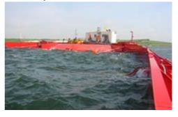
The Wave Dragon structure is stationary set up to face the predominant wave conditions. The turbines are the only moving parts.
