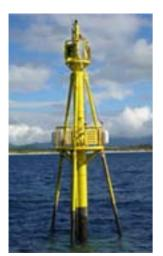
using large specialised buoys anchored to the sea These buovs bed. convert the wave energy into electricity via a number of 'power take-off systems'. Offshore trials were first conducted off the coast of New Jersey, USA from 1997, and the company are currently moving towards the commercial application of these buoys. The first 50kW 'PowerBuoy' has recently been installed in Hawaii.
