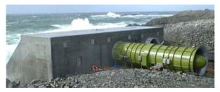
world's first commercial scale wave energy converter, located on the coast of Islay in the Highlands of Scotland. It is the smallest of Wavegen's shoreline energy modules, and generates 0.5MW of power for local communities. There are now plans for Wavegen to install a LIMPET style generator on the Faeroe Islands.
