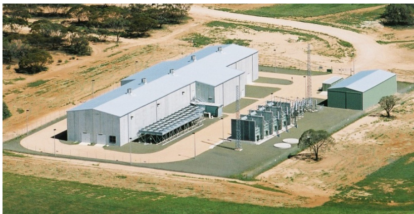
Figure 2.1 Murraylink HVDC Light, Berri Station (220MW)
