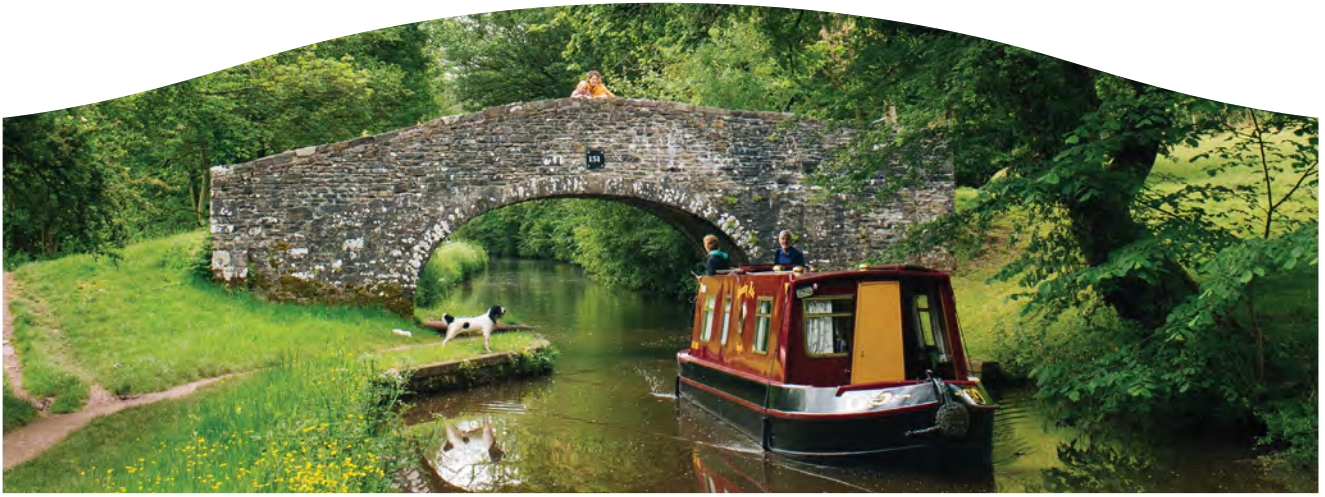
Above: Monmouthshire & Brecon Canal
