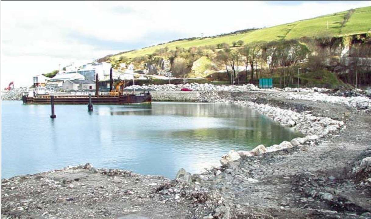
Harbour improvement works at Glenarm were licensed under FEPA.
