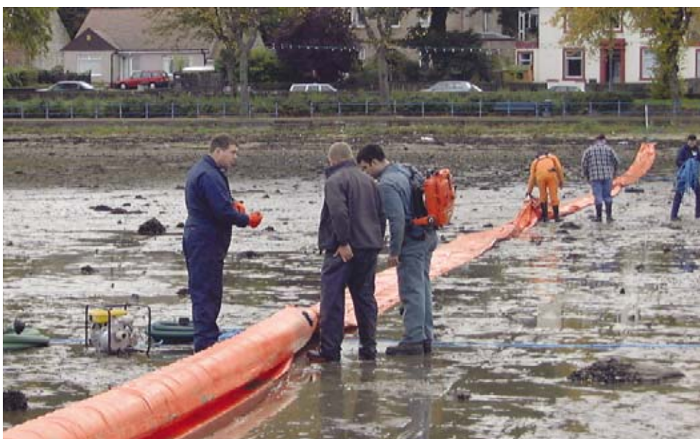
Laying a boom to trap oil following a coastal pollution incident
