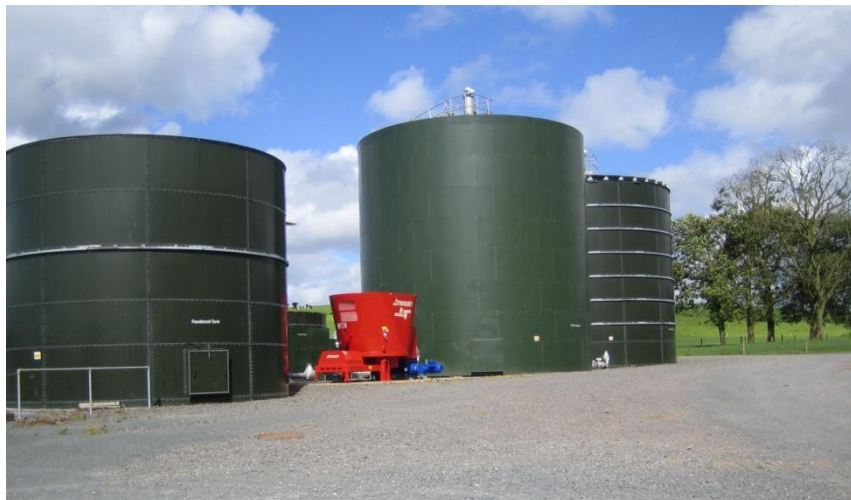
Figure 1: Photograph of AD plant at AFBI (digester tank centre)
