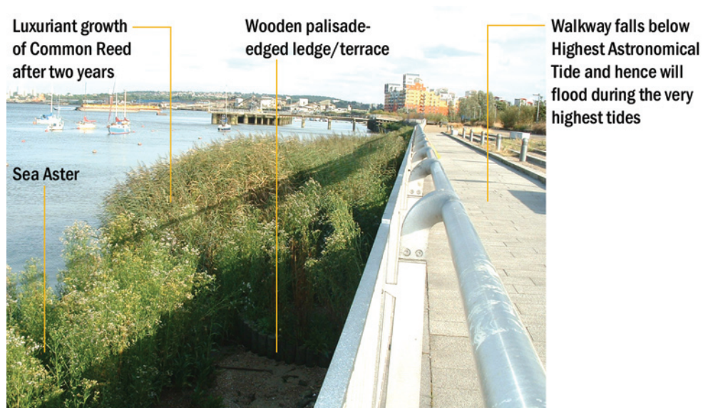
Eastern wall, Greenwich Peninsula, London: Site 2, south end, three years after implementation
