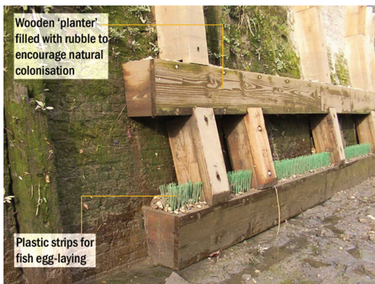
Deptford Creek, London: Timbering to river wall
