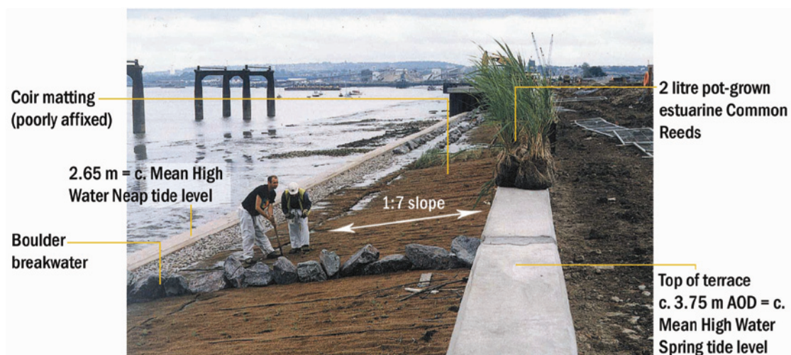
Eastern wall, Greenwich Peninsula, London: Site 2 during construction
