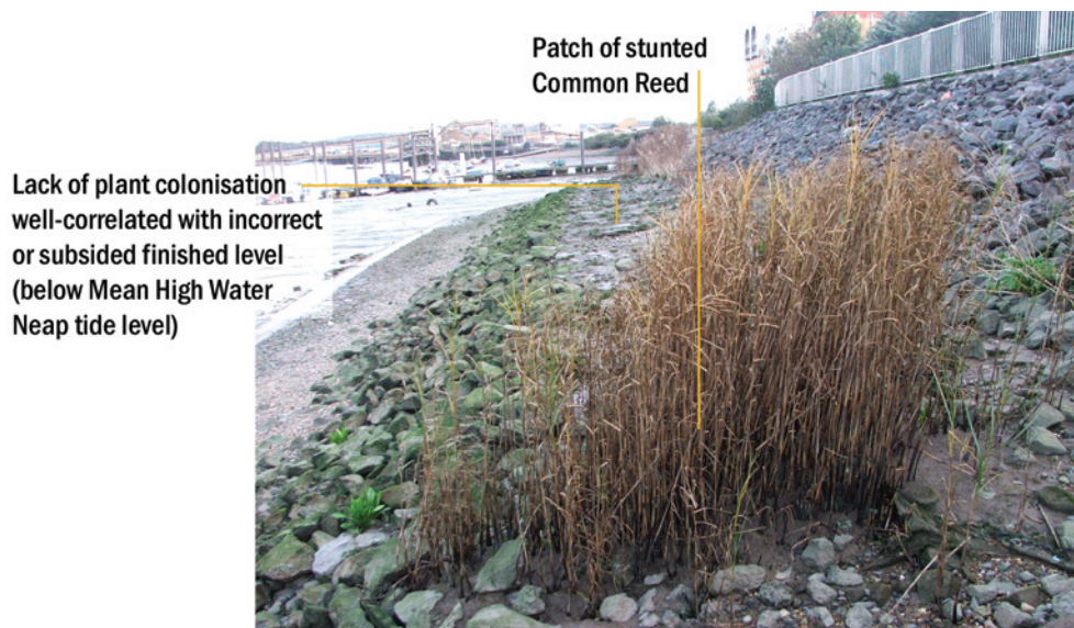
Greenwich Peninsula, London: Site 1 from north, eight years after implementation (winter)
