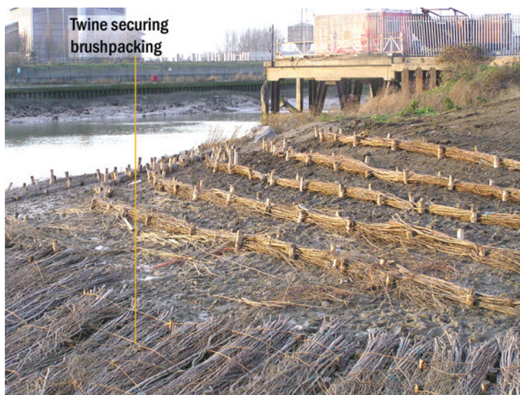
Barking Creek at Barking Barrier: Fixing detail of brushpacking
