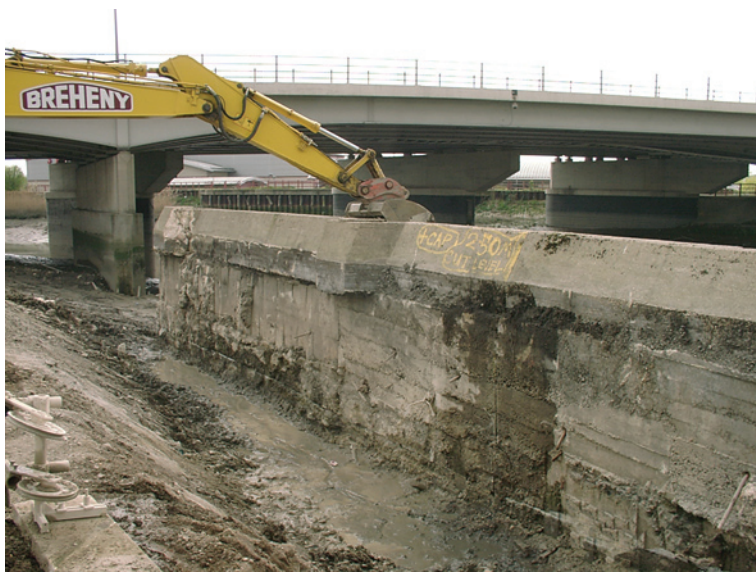
Barking Creek at A13: Demolition of river wall
