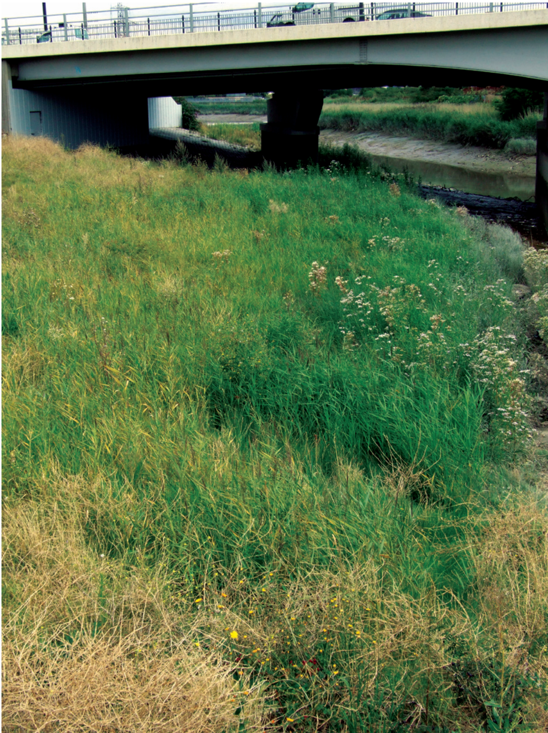
Barking Creek at A13: Vegetation establishment after 14 months
