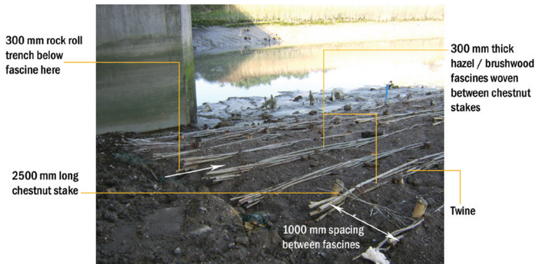
Barking Creek at A13: Details of fascine installation near bridge
