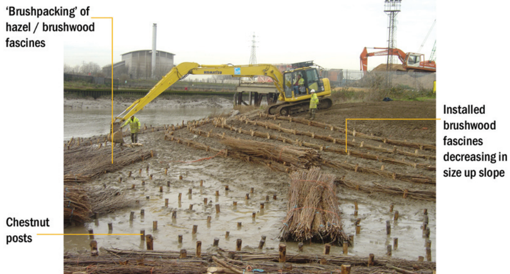
Barking Creek at Barking Barrier: Delivery of brushwood bundles
