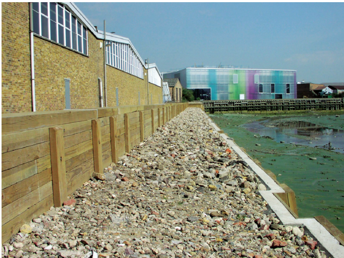
Top of river wall along Deptford Creek, London
