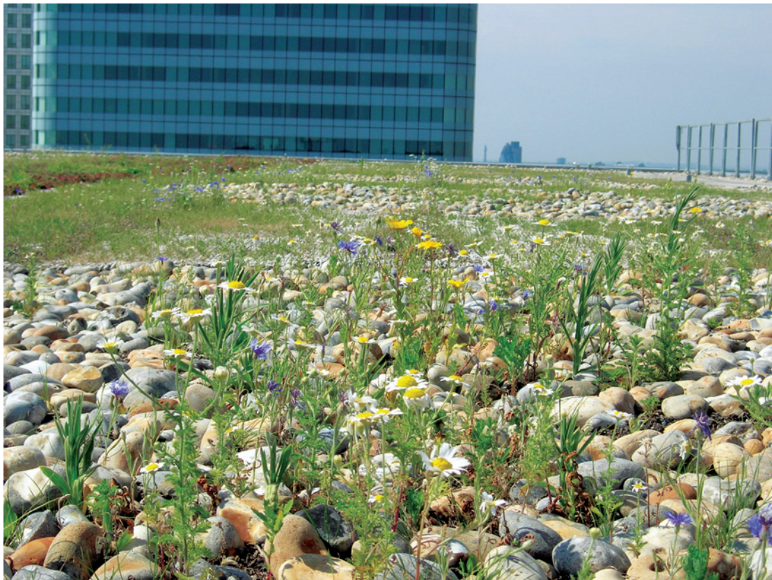
Low-nutrient eco-roof in London
