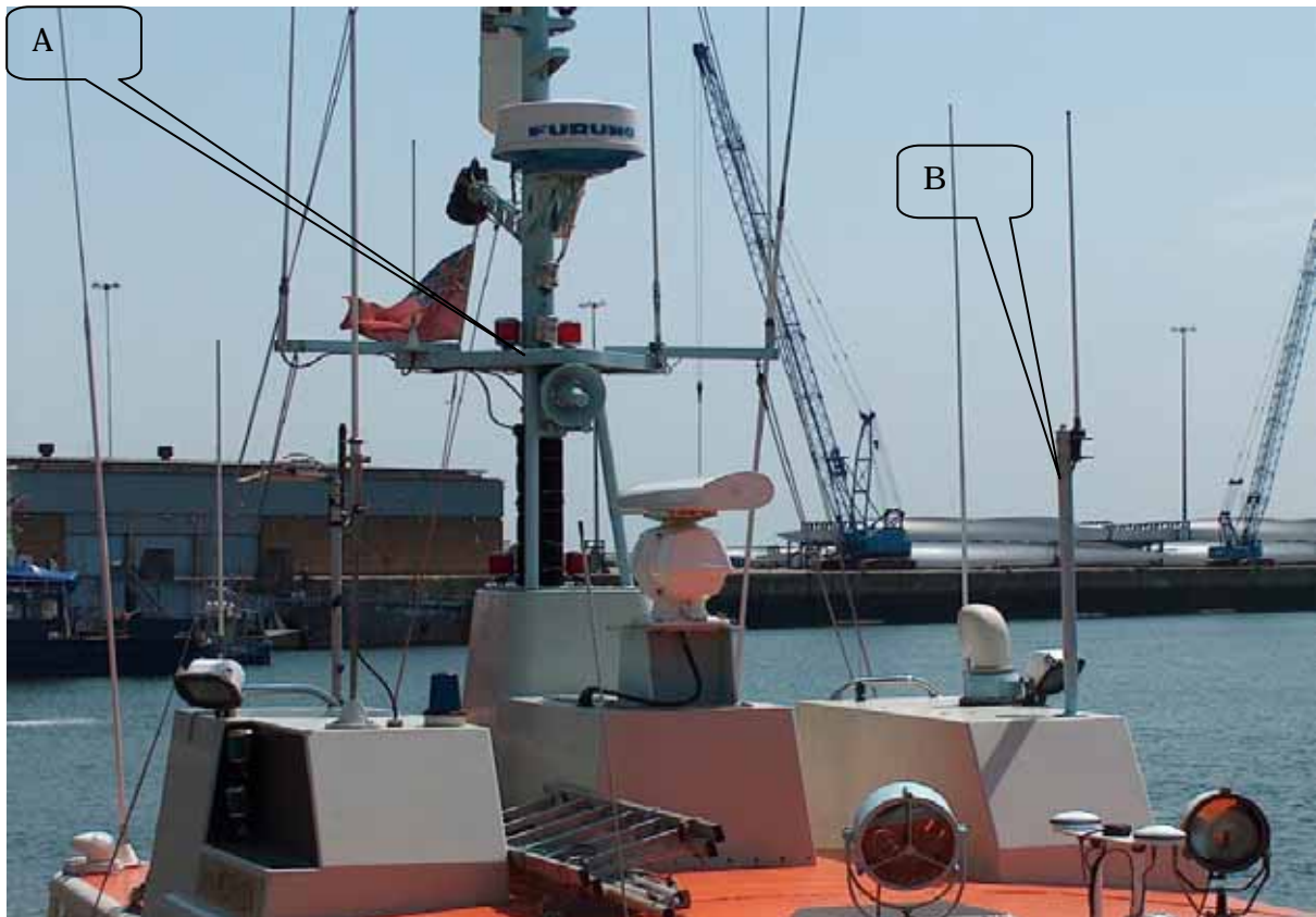
Figure 27: “MORVEN”: View from starboard bow looking aft. The main (X-Band) scanner is centrally mounted. The signal mast ‘A’ and the 50mm pipe stanchion ‘B’ are producers of spurious echo sectors. Note “Radar Absorbent Material” (RAM) – in this case Engine Sound Insulating Foam; black in colour was wrapped round the mast to decrease effects. Although not very apparent from the angle of this photograph; it should be noted that the two mast support struts are angled aft at the top and therefore deflect radar beam interceptions upward.
