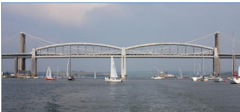
Royal Albert and Tamar Bridges joining Devon and Cornwall (Chart point 1)
