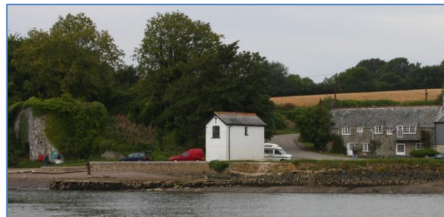
Halton Quay and the smallest chapel, with the remains of the lime kilns on the left. (Chart point 7)
