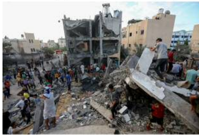
A residential building in Khan Younis was struck on Oct. 17 Yousef Masoud for The New York Times
