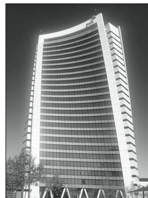
PricewaterhouseCoopers Building In Johannesburg, South Africa. Photo: TapticInfo – flickr.com (CC BY-SA 4.0)
