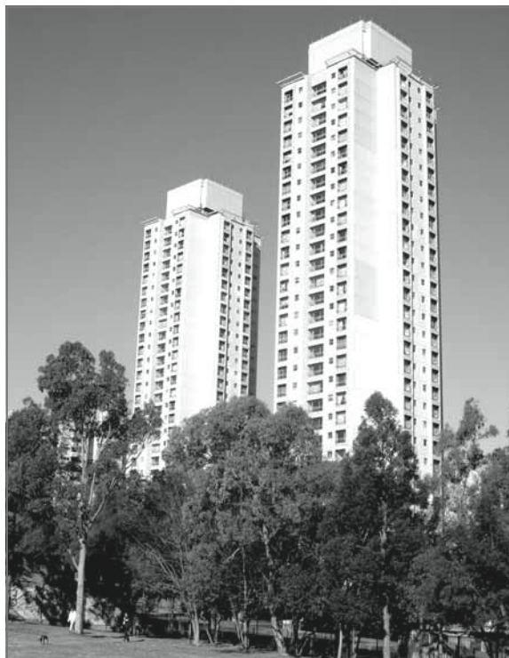
Public Housing Towers, Waterloo, Sydney. Photo: J Bar – Wikimedia Commons (CC BY-SA 3.0)
