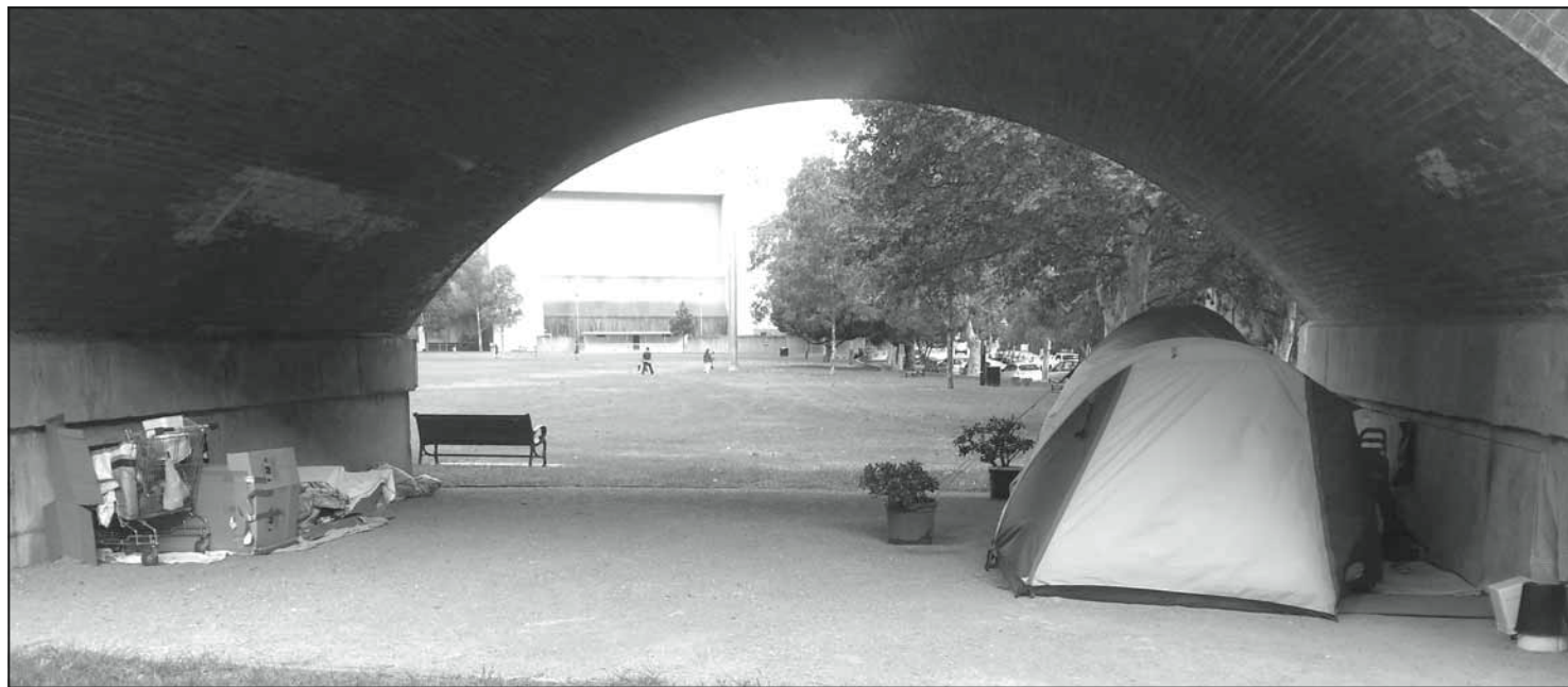
One of the many arches that are part of the aqueduct that goes over Wentworth Park Glebe. These arches are filling up with the homeless while just a short distance away public housing remains empty.
