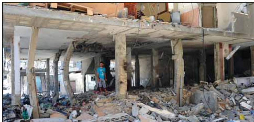
A Palestinian resident walks amongst the rubble of a destroyed building in Gaza. Photo: United Nations Photo – flickr.com (CC BY-NC-ND 2.0)
