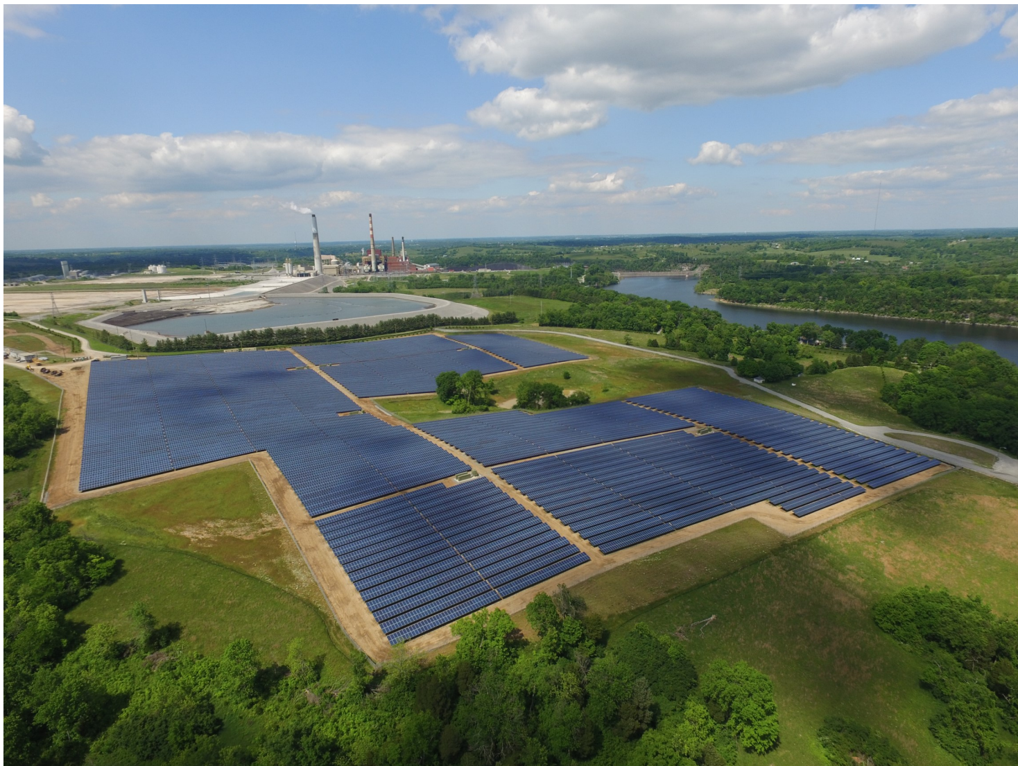
Aerial view of E.W. Brown Solar Facility. Photo courtesy of LG&E-KU.
