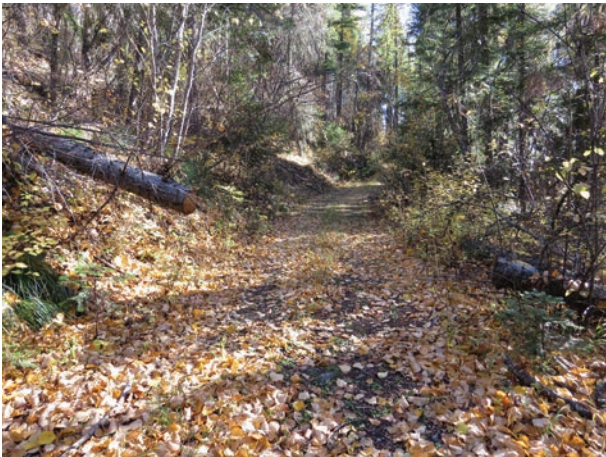
Fig. 10: Clearing of road 5392Y behind its closure device.
