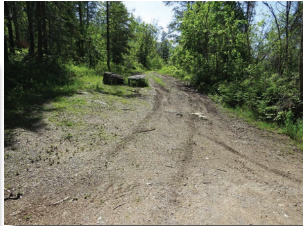
Fig. 11: 6/17/22 photo of road closure 5392Y.
