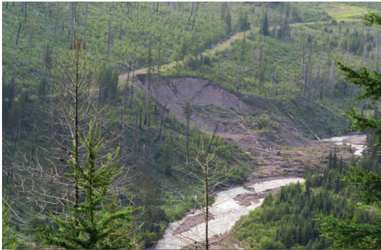
Water collecting in the ditch of this closed road contributed to mass failure into Sullivan Creek, a key bull trout spawning stream.
