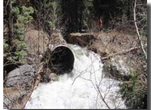
Flathead NF photo of a 4' plugged culvert putting the Emery Creek Road into trout habitat!
